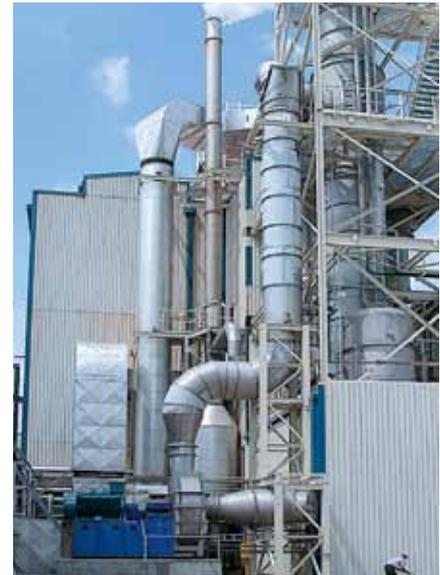
Single-effect falling film evaporation plant with mechanical vapour recompression for wheat starch effluent, evaporation rate: 17,000 kg/h
