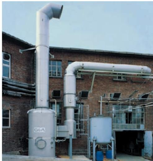
*Single effect continuously adjustable Venturi scrubbing plant type U for washing out dusts
