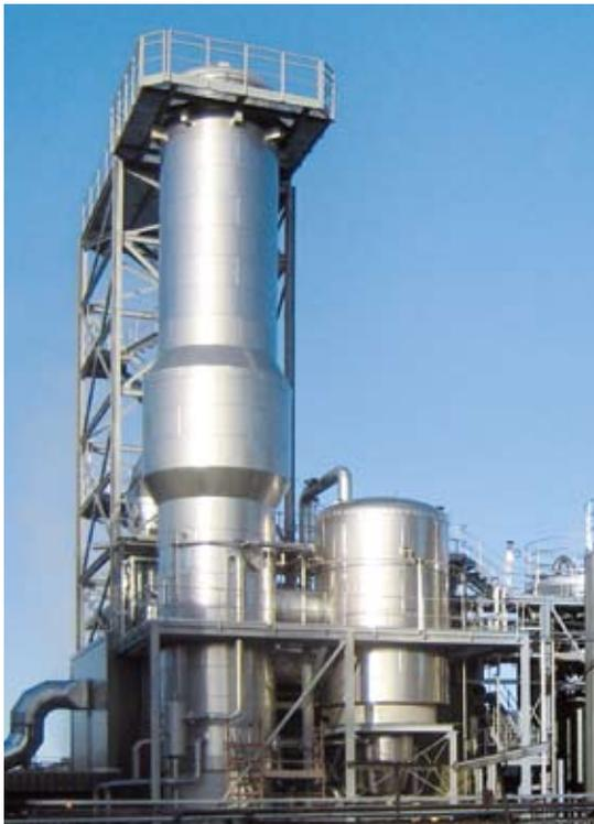
Single-effect falling film evaporation plant with mechanical vapour recompression
