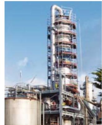
*Energetically optimized IPA distilling plant for typical capacities with feed rates of 20 to 100 t/h*
