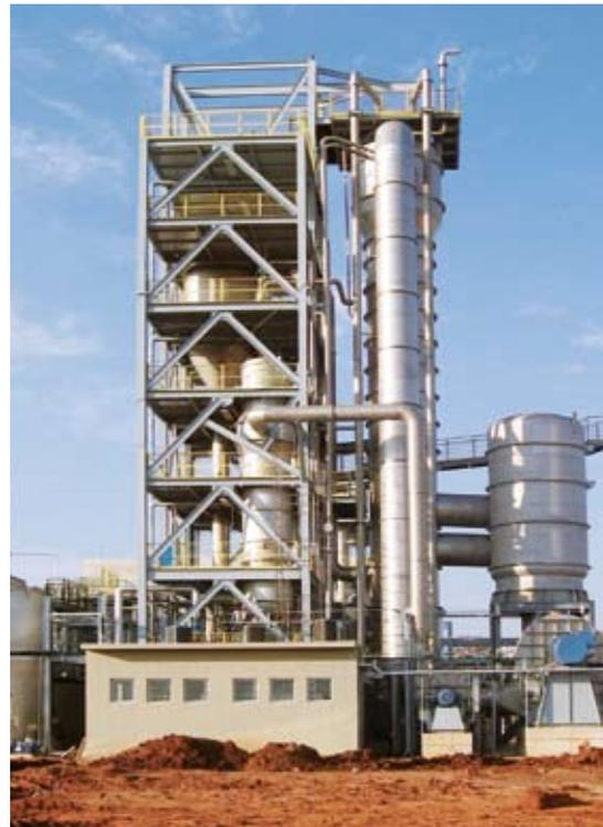
Evaporation plant with 2 fans for mechanical vapour compression and a forced circulation evaporator as finisher
