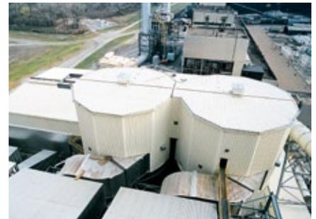
*Large SDA's clean the flue gas from a 550 MW<sub>e</sub> coal fired power plant in the USA.*
