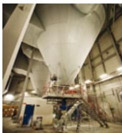
Bottom of SDA with flue gas inlet and outlet duct and product discharge.
