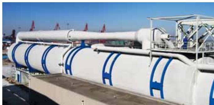
Evaporators are used in the MED- and MSF-processes. These operate under vacuum in order to achieve the best performance rate. In all cases, the vacuum is created using multi-stage steam jet vacuum pumps.
