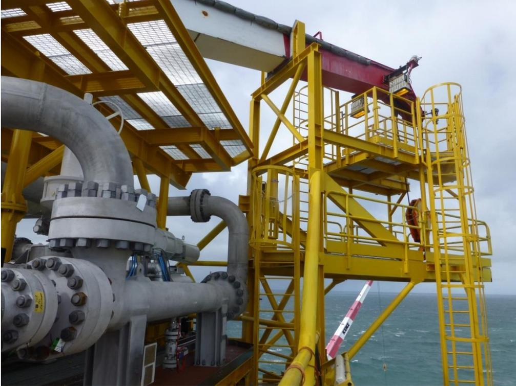
*GEA designed, manufactured and delivered a gas jet compressor system for an offshore platform in the North Sea.*
