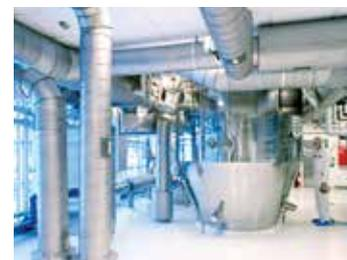
PHARMA-SD™ type PSD-4 drying chamber and HVAC ducts.
