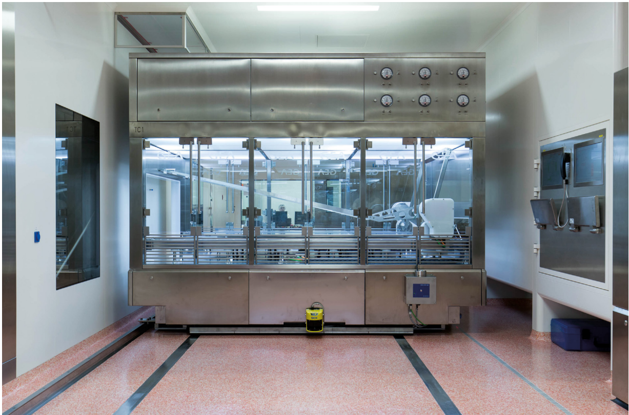
Production Line with ALUS® Cross moveable Transfer Cart.
