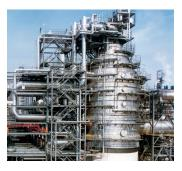
Thermocompressor with variable flow for a multi-effect distillation unit for a seawater desalination plant with a capacity of 800 t/h of distillate.
