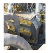
An important pre-requisite for Carbon Capturing is **Flue Gas Pre-treatment** to ensure the long-term stability of the Carbon Capturing system. **GEA SETO** technology line offers various solutions to remove solids, aerosols, sulfuric and nitric oxides and more.
