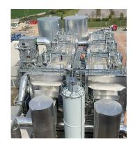
The current state-of-the-art process for large scale  ${\bf Carbon\ Capturing}$  is by chemical absorption with amines. GEA offers amine-based  ${\bf CO_2\ capture\ plants\ of\ various\ sizes}$  under the  ${\bf GEA\ CEBO\ line}$ , allowing for  ${\bf CO_2\ capturing\ from\ very\ diverse\ exhaust\ gas\ compositions}$ .
