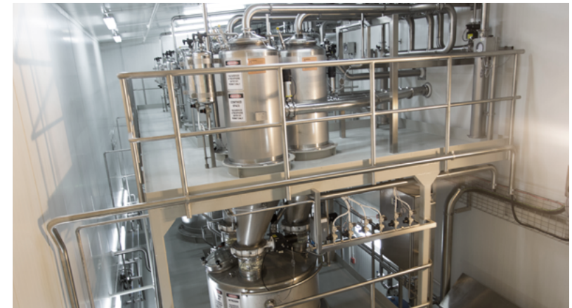
Pre-gassing system for modified atmosphere powder packing lines (MAP)
