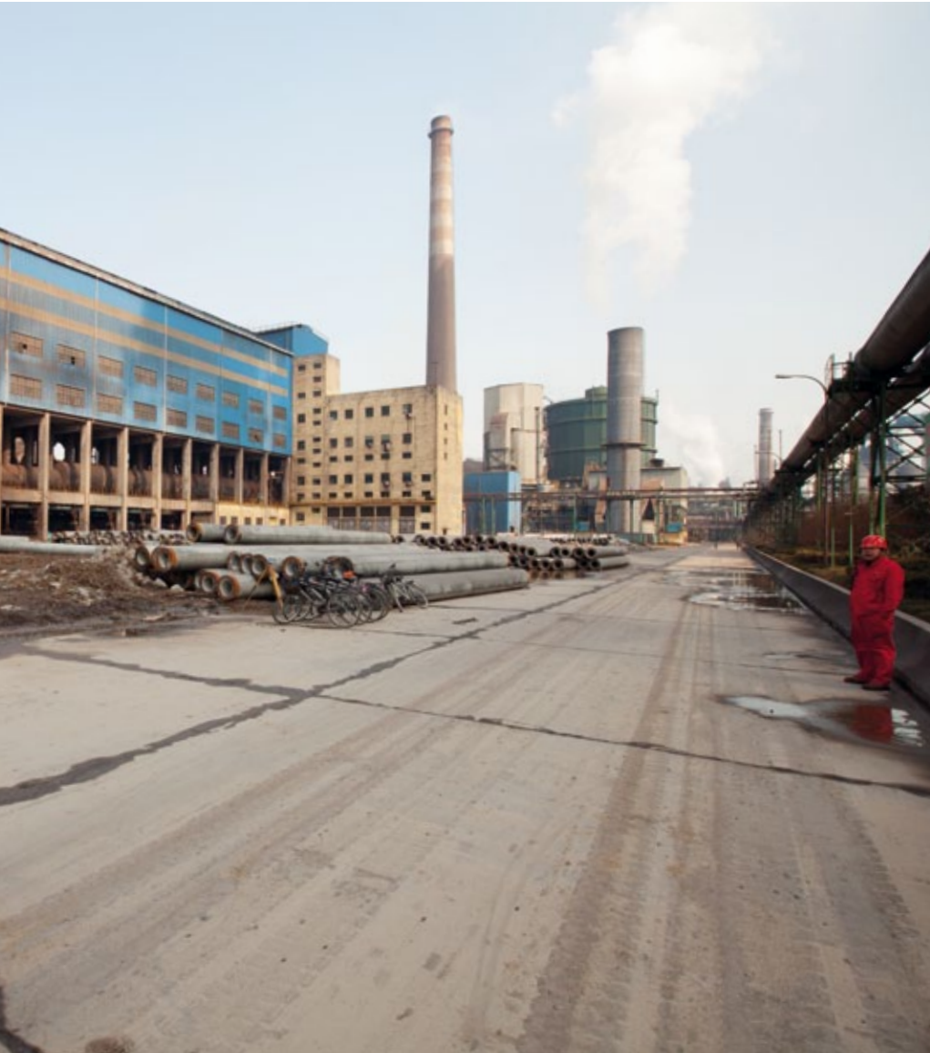
360 m 2 sinter band installation (left) with GEA Niro spray dryer absorber, bag filter and new stack (background)
