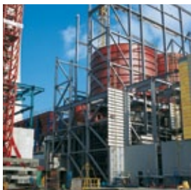
Left: Erection of an SDA plant in Denmark.
