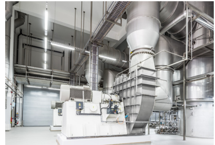
Evaporator with MVR fan
