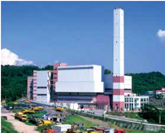
A Taiwanese waste incineration facility with two GEA Niro SDA systems, 2 x 300 TPD.
