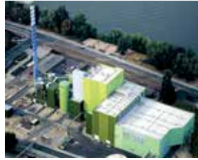
Left : A GEA Niro SDA system at two waste incineration lines in Germany, 2 x 300 TPD.
