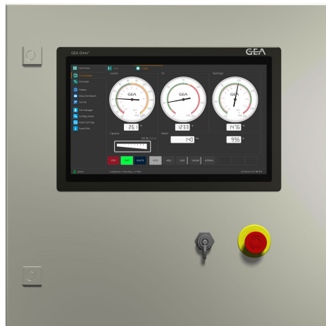
Fig.10: GEA Omni exterior view without indicator lights
