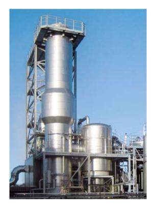
Single-effect falling film evaporation plant with mechanical vapour recompression Evaporation rate: 40 t/h After the biomass separation and further treatment steps, the fermentation solutions are concentrated in falling film evaporators up to a solid content of 50 % DS. The further concentration and crystallization then takes place in forced circulation evaporators and in crystallizers.
