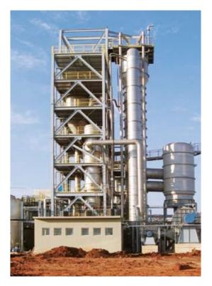
Evaporation plant with 2 fans for mechanical vapour compression and a forced circulation evaporator as finisher Evaporation rate: 67 t/h
