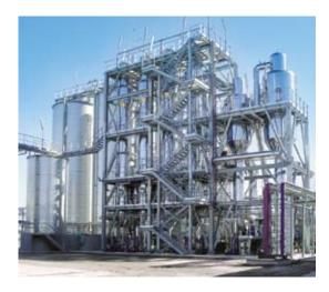
4-effect falling film/forced circulation evaporation plant with thermal vapour recompression for fermentation waste water Evaporation rate: 31 t/h
