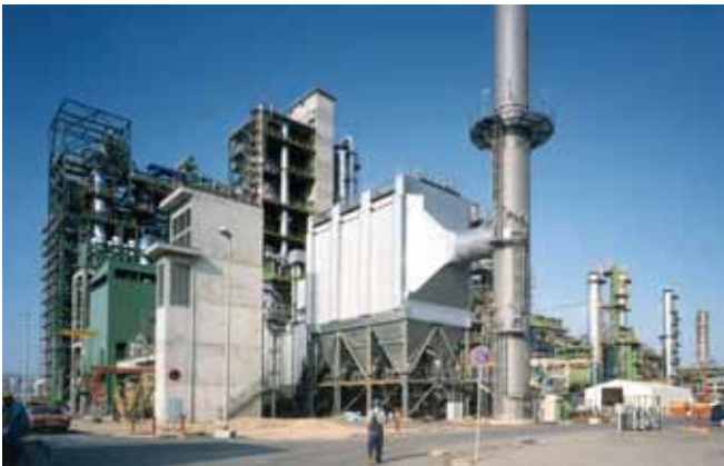
Installation of a three-field ESP ...
