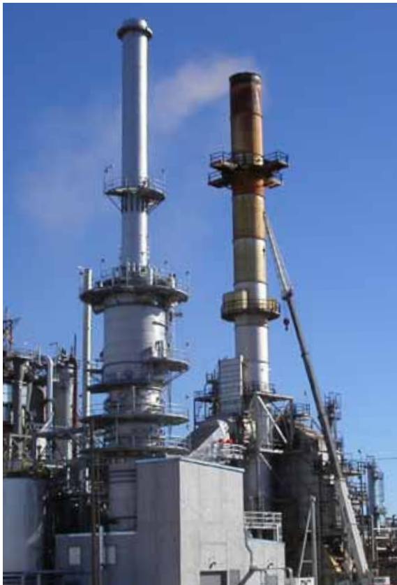
EP-Absorber with soda ash reagent storage, pump house and control building. Reference example: Tesoro Corporation, Tesoro (USA)
