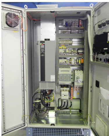
Fig.14: GEA Omni™ control cabinet interior view (frequency converter installed in control cabinet)
