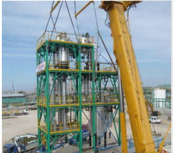
*For small-scale applications, a skid-mounted modular concept has been developed to recover high quality process condensates and separated (disposable) solids, meeting the critical reliability and availability requirements of a power plant.*
