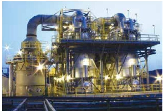
*Wet gas electrostatic precipitator for nickel smelter*
